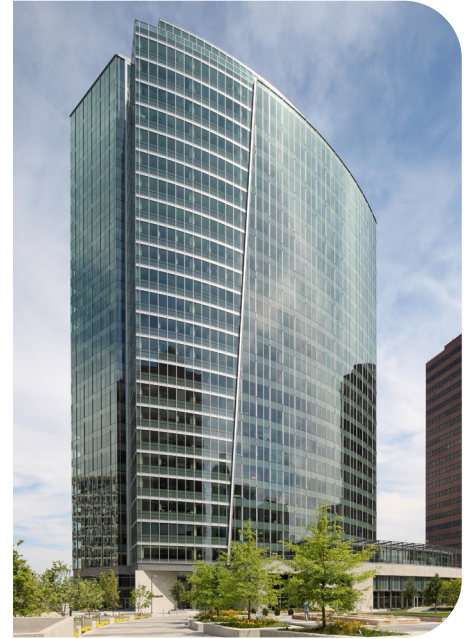
City Center Plaza incorporates a wide range of environmental features, including the use of Solarban ® 70 glass, which, despite its clear glass appearance, has the industry’s highest light to solar gain (LSG) ratio.
